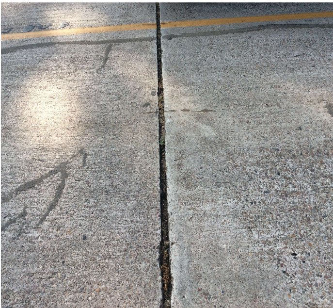
PHOTO 1 Description Joints need to be cleaned and refilled
