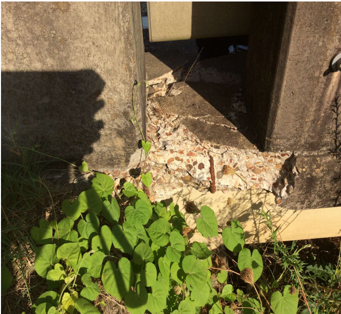
PHOTO 1 Description Damage to curb and overhang left side at bent 4
