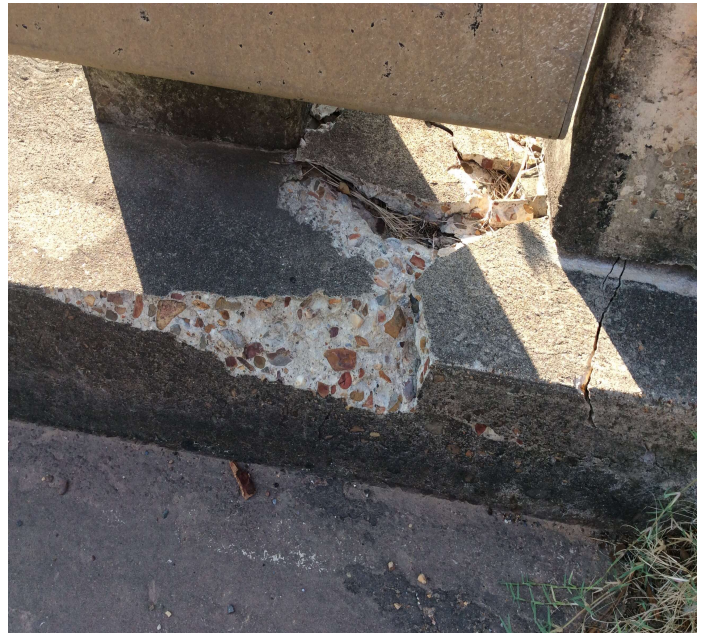
PHOTO 2 Description Curb and overhang at bent 4 left side damaged
